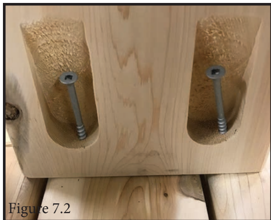
Figure 7.2 Shows how the large pockets allow for angling the screws to ensure alignment into the deck boards.
