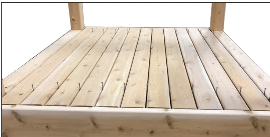
Figure 7.1 Shows how to use the screws for spreading out deck boards with even spacing.
